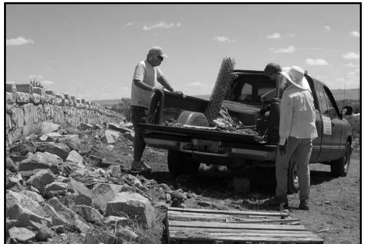
NMJHS volunteers rebuild a cemetery wall.
